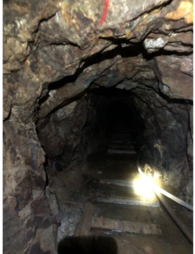
Photo 3: Old railway sleepers still in place in the floor of the main access adit.
